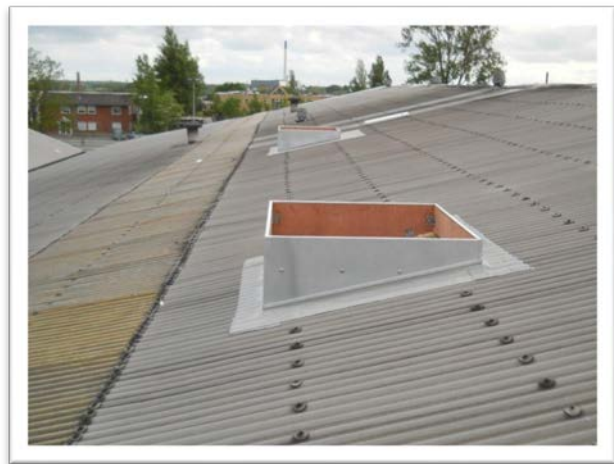
Example of base on sloping roof
