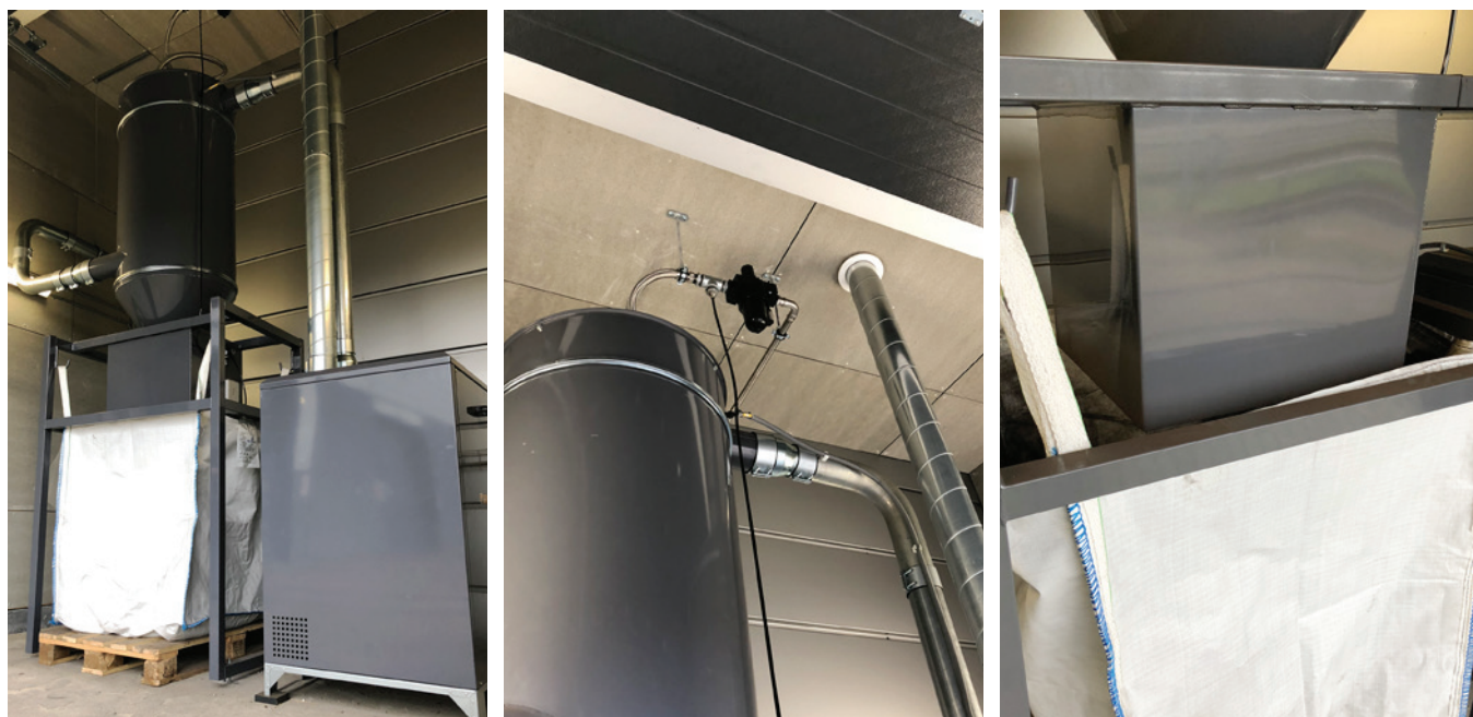
HVU Solo. Stand-alone side channel blower module.
